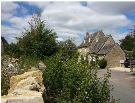
Obstructed visibility to the left from existing boundary wall (measured >2.4 metres back from edge of carriageway)
